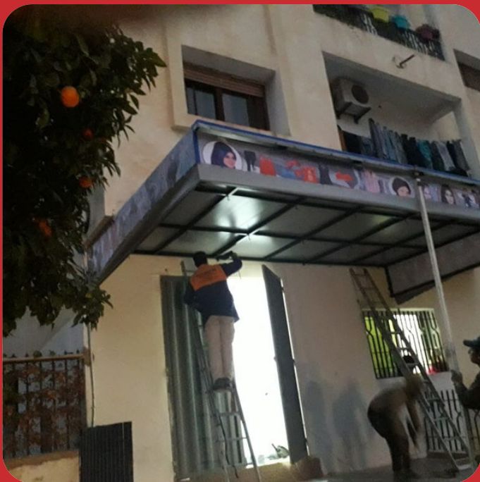
Suni's clothing shop under construction
